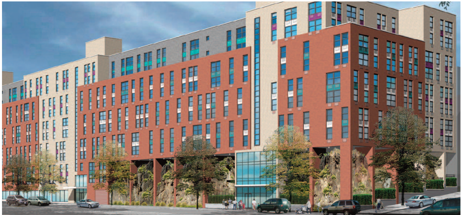
The Roscoe C. Brown apartment building will incorporate an existing rock outcropping into the structure.
